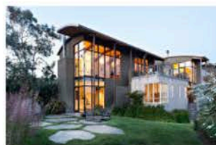
The View House in the Oakland hills, designed by David S. Wilson, AIA, closes off the front of the house to the busy street with plaster, steel and concrete and opens it to the landscape with two stories of glass.
